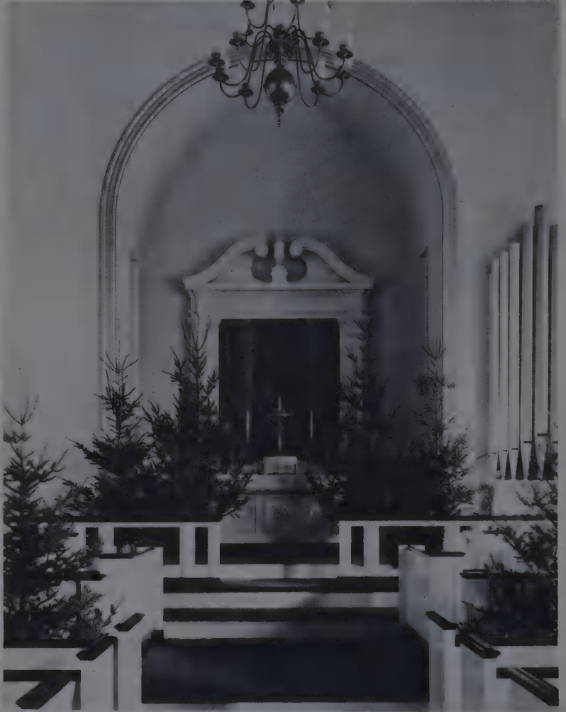
Saint Paul's Church, Millersville, Pennsylvania
