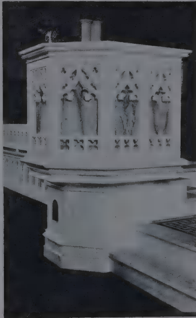
The pulpit in Trinity Church, Canton, Ohio Gothic—Carrara marble with Breccia marble panels
